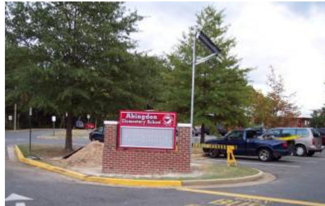
LED Retrofit, Arlington County Schools
