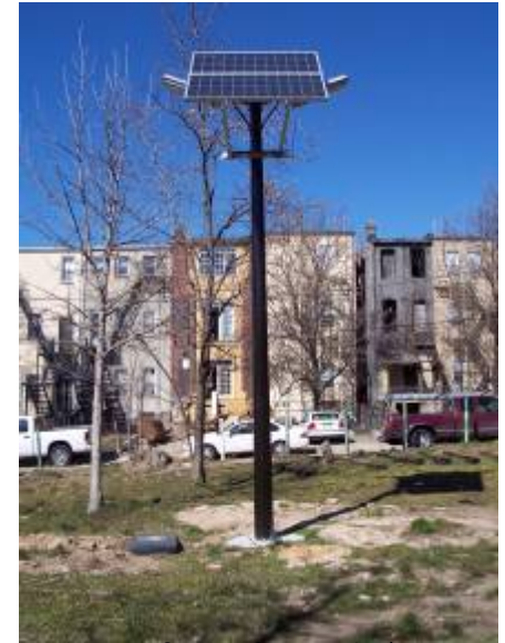
Motion Sensor Security Lighting Solar Powered LED Street Lights Greenmount West, Baltimore
