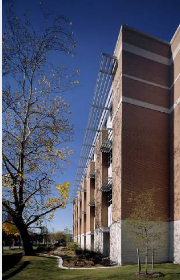
South Facing Solar Shading Screens
