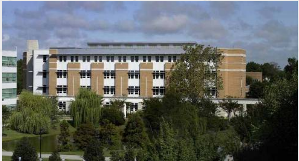
View of Roof Top Daylight Monitor
