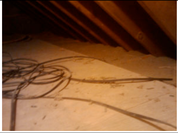
Low insulation in small attic
