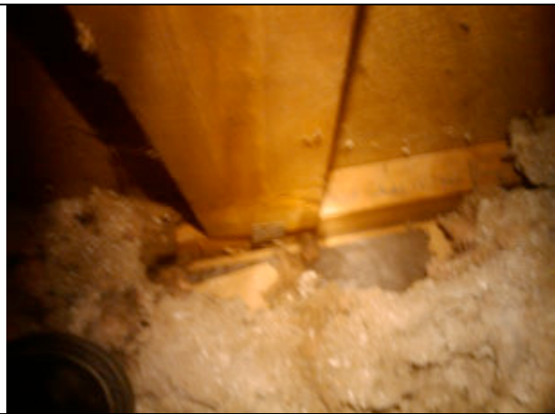
Attic knee wall without a sealed air barrier
