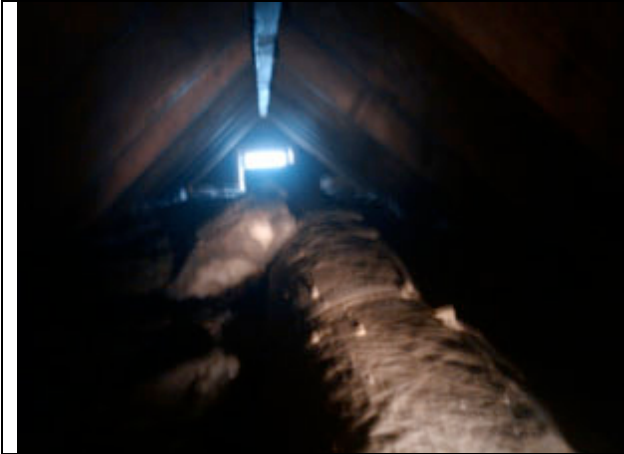
Small attic above finished room
