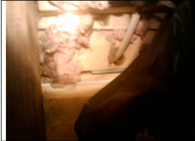
Seal top plates of walls and wire penetrations
