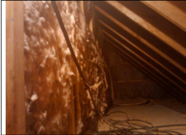
Attic knee wall without a sealed air barrier
