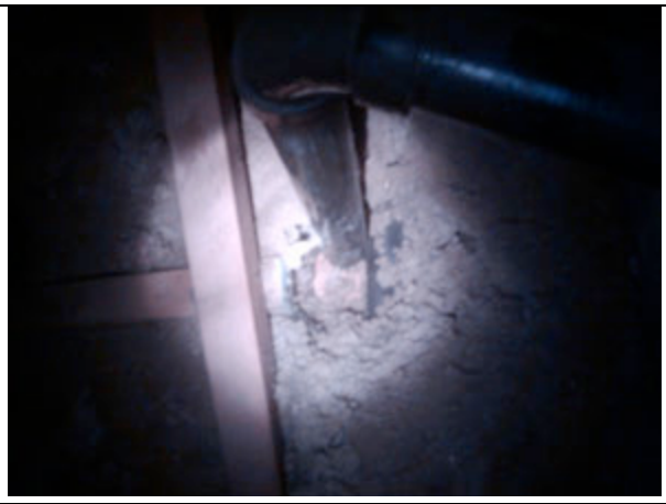
Low insulation in small attic
