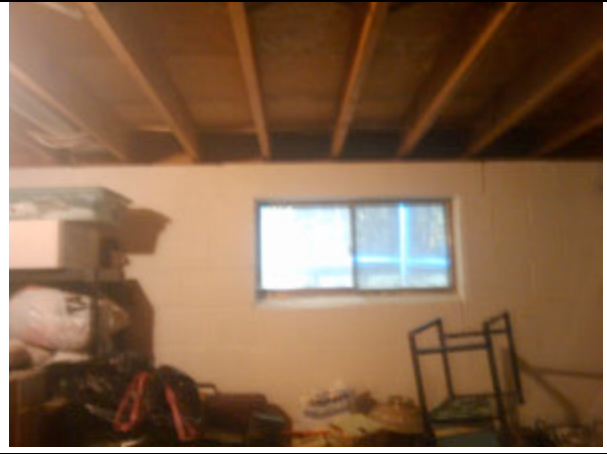
Air seal and insulate band joists
