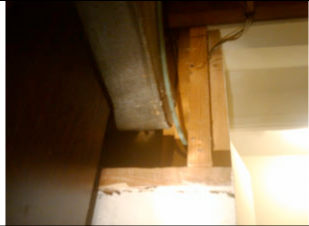
Open duct chase needs air barrier and sealing
