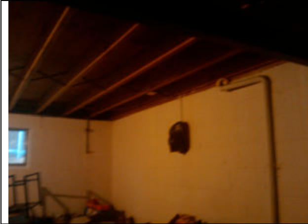
Air seal and insulate band joists
